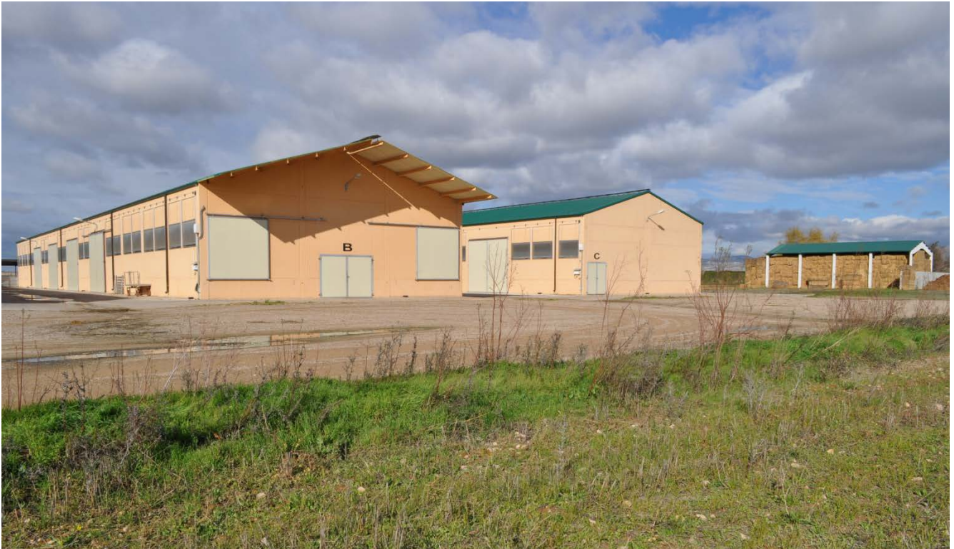
Figure 4. Lamb reception (B) and fattening (C) barns. Straw barn in the background.
