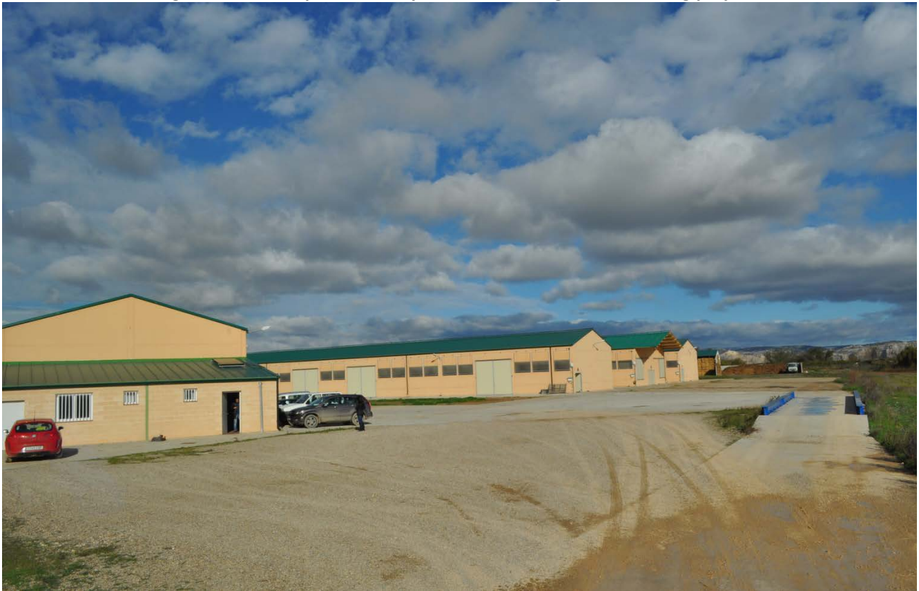
Figure 3. General view of the FyN lamb complex, with truck scale, straw barn and manure stocking area in the background.
