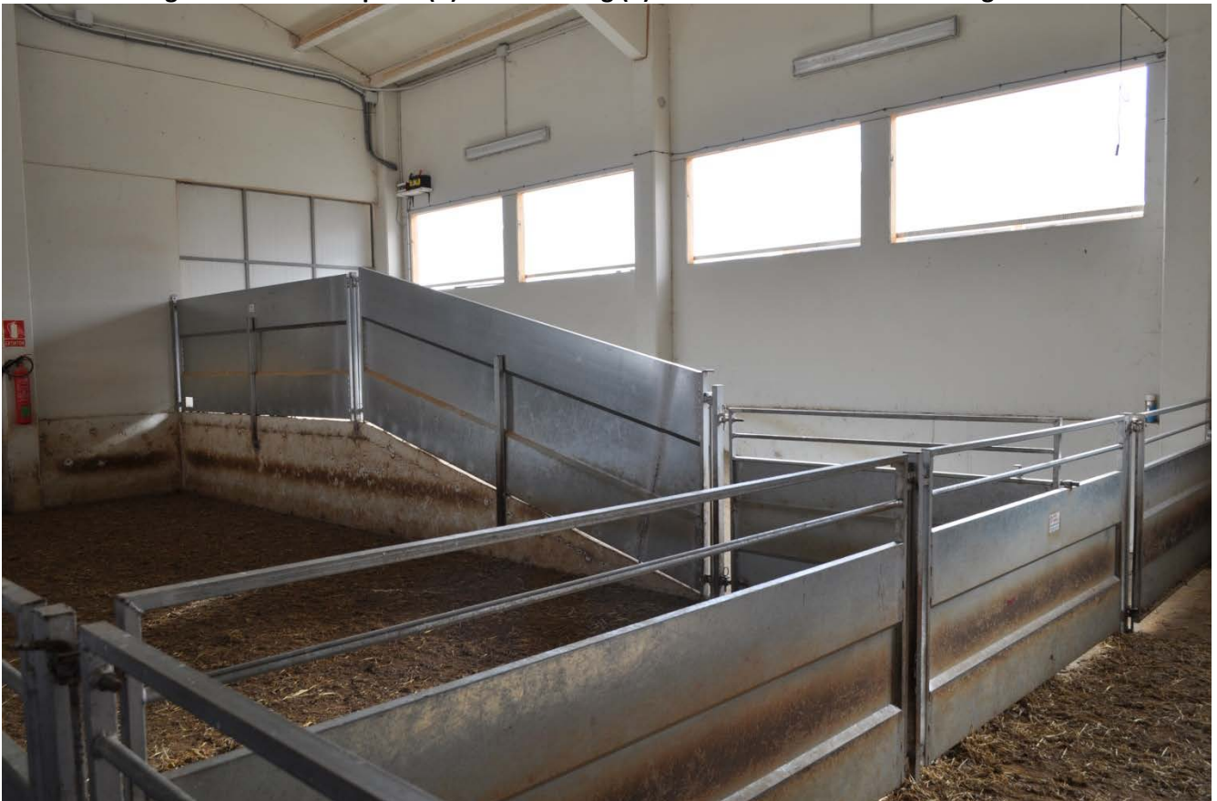
Figure 5. Loading bay and ramp inside the lamb reception barn B.
